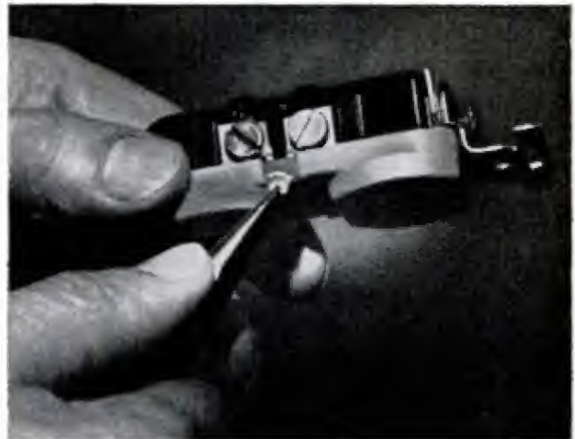
REMOVING LINK between terminals on one side of upper duplex outlet splits the circuit so the outlet can power two lights independently of one another
